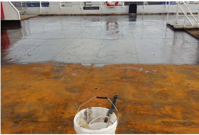
Solvent-free primer-finish coating for highly saline environments, applicable directly on rust
